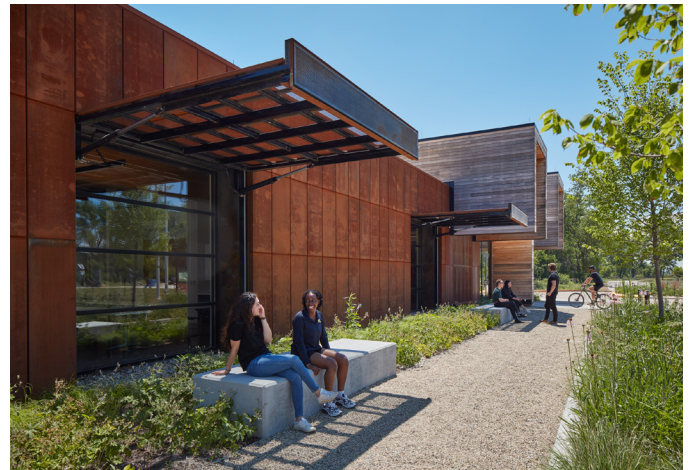
Operable hangar doors provide shade while protecting birds from reflections in the building’s windows.
